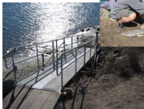
Duke Energy Corp. Plant
